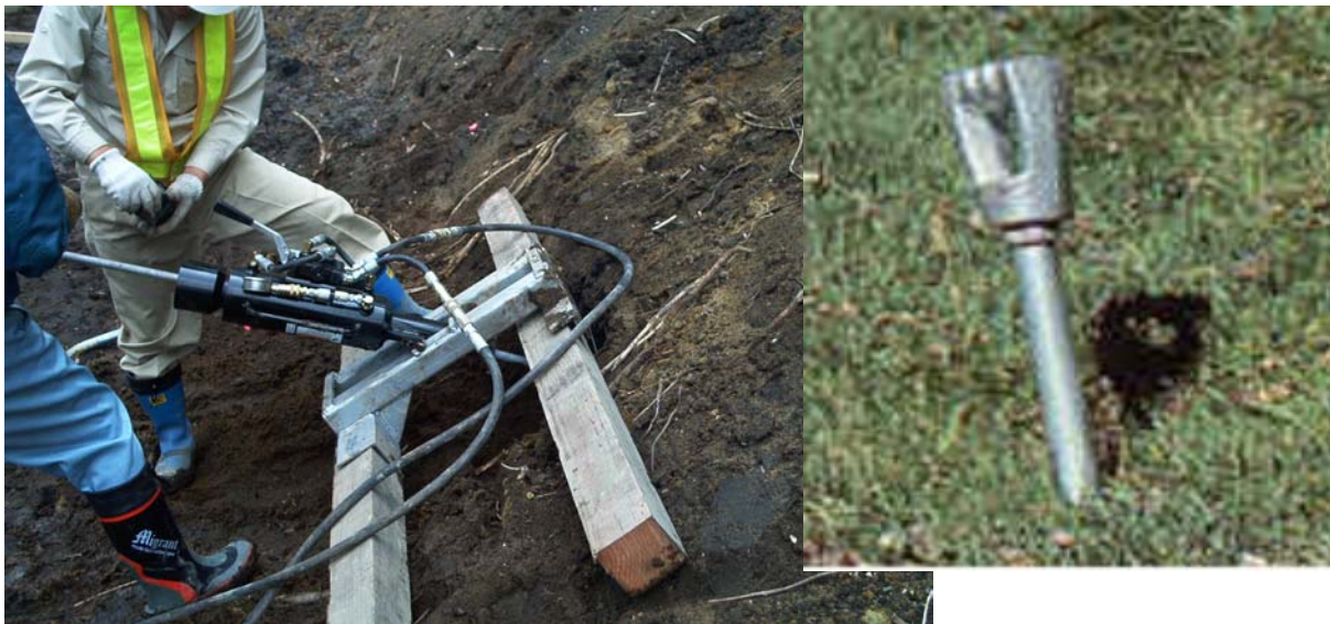
Load locker base is placed on timbers in soft soil, and finished anchor with eye nut installed.
