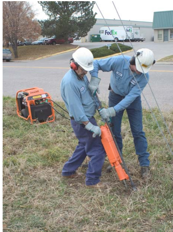
Top of anchor rod at grade, and Adapter Setting Bar (ASB) being installed.
