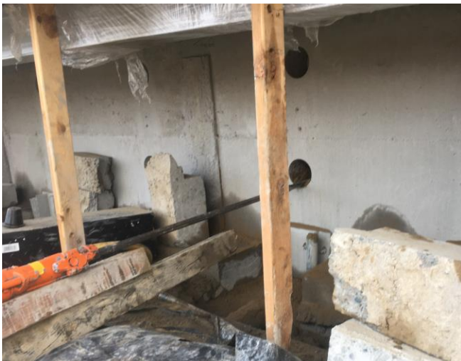
Low Overhead Clearance: Pre-drilling holes in the dense ground prior to installation of the Manta-Ray MR-4. Overhead clearance of 48".
