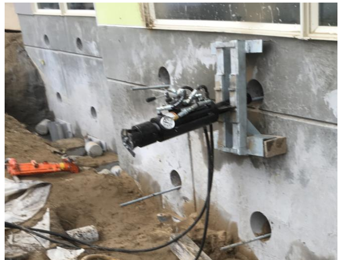
Load Test: Tieback lock-off equipment in place and ready. Tiebacks tensioned to 10 kips and locked off. Note the pin piles and underpin brackets at the footing level.
