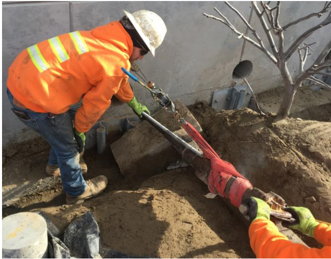
Manta Ray Installation: Installing the Manta-Ray MR-4 with a 90# jackhammer, using a come-along to apply crowd.
