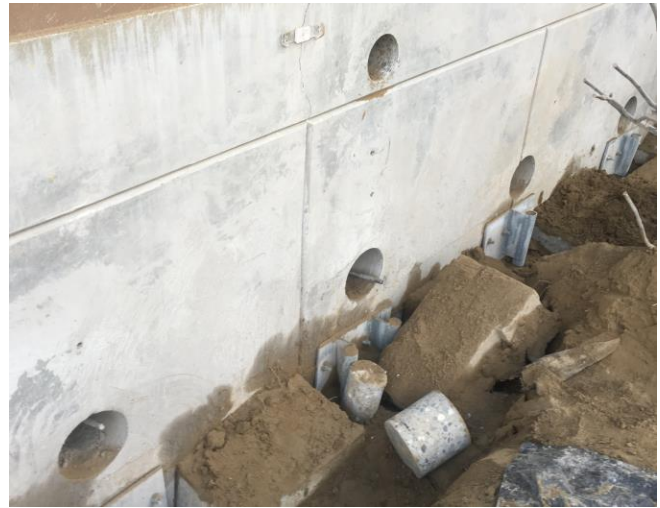
Foundation Core Drilling: Holes cored in the foundation to allow installation of the Manta-Ray MR-4
